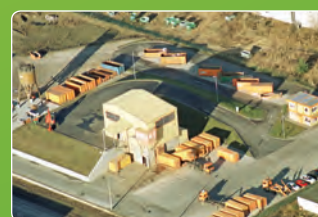
Waste Transfer Station Güstrow
