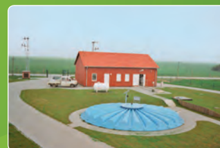
Sewage Treatment Plant Breege
